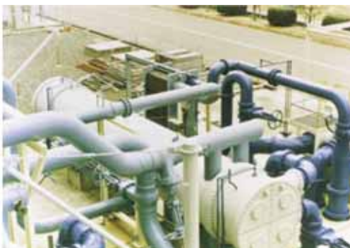
The shell and tube was growing prohibitively inefficient
