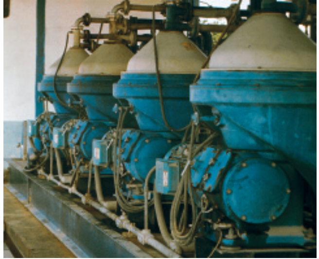
GT separators - the heart of a successful fuel treatment plant.
